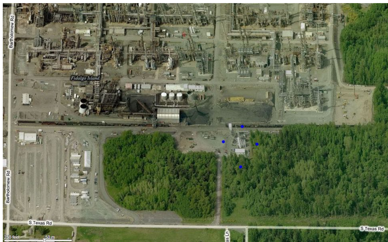
Figure 2-2 A view of the Air Liquide facilities (surrounded by blue dots), with the PSR refinery to the north (photo from bing.com).
