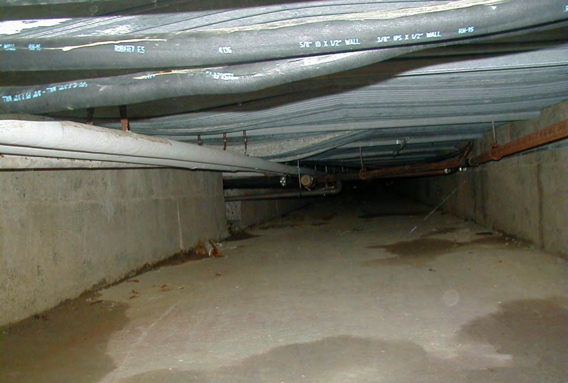
Tunnel is air duct for school
