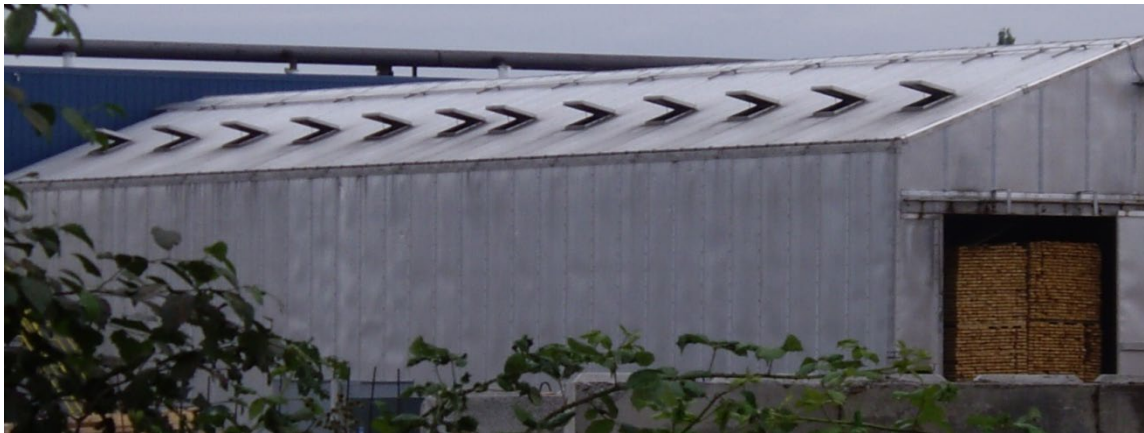
Figure 2-9 Dry Kiln at Cycle End
