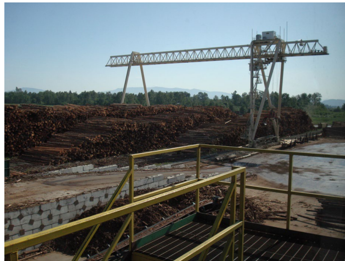
Figure 2-4 Log Storage and Crane
