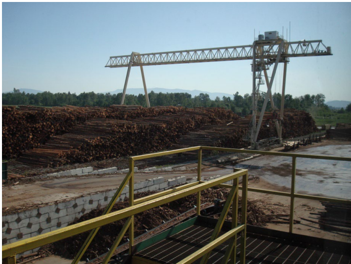
Figure 2-4 Log Storage and Crane
