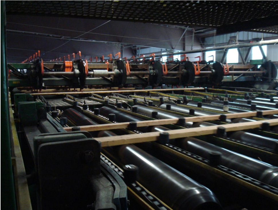
Figure 2-6 Lumber Sorting Line
