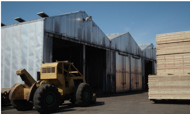
Figure 2-10 Dry Kilns Ready to be Loaded
