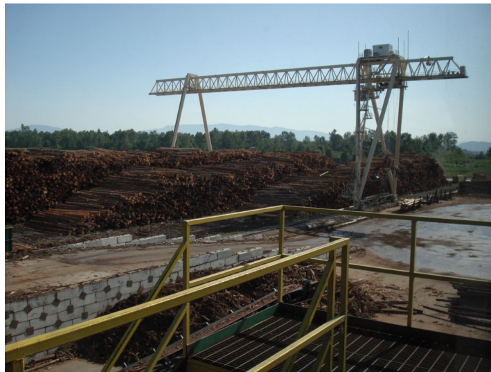
Figure 2-4 Log Storage and Crane
