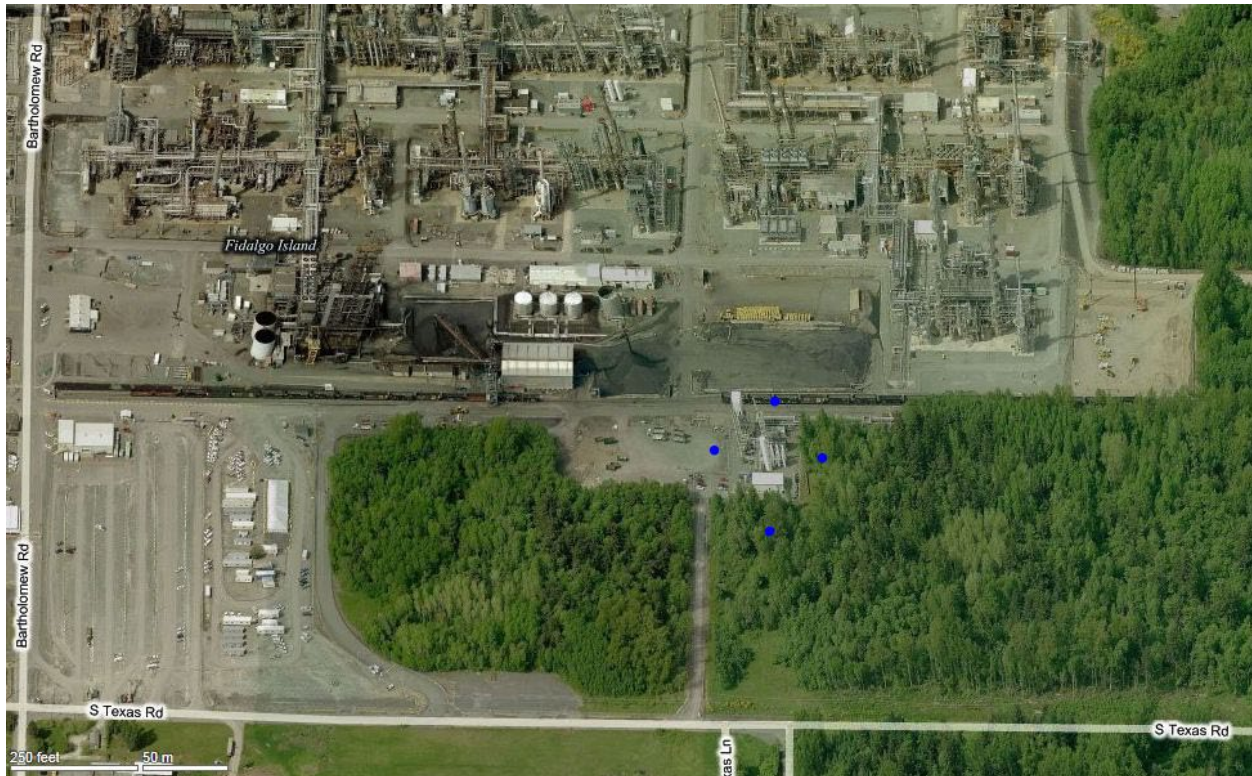
Figure 2-2 A view of the Air Liquide facilities (surrounded by blue dots), with the PSR refinery to the north (photo from bing.com).
