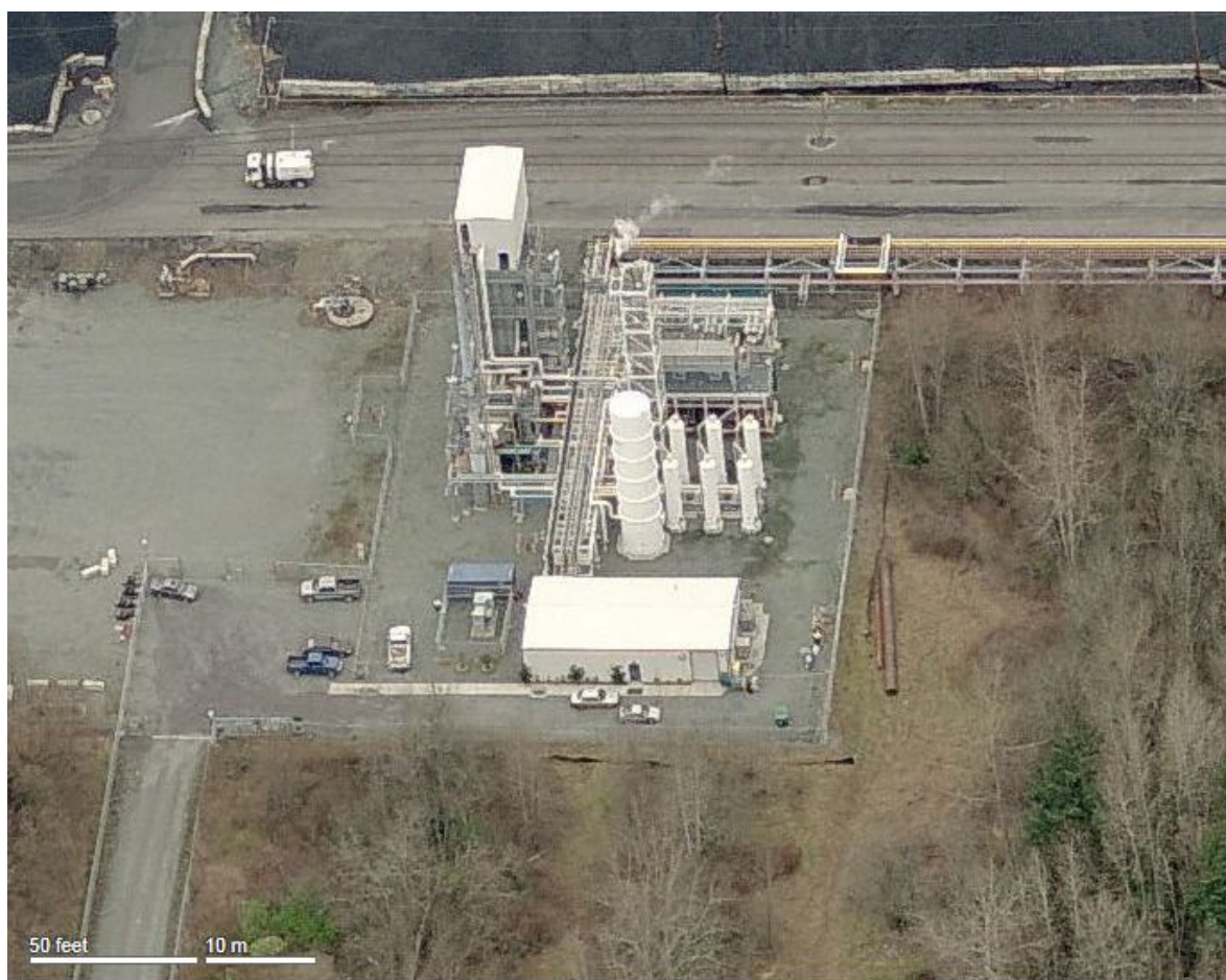
Figure 2-1 An aerial photograph showing the Air Liquide facilities at Anacortes, WA (photo from bing.com).
