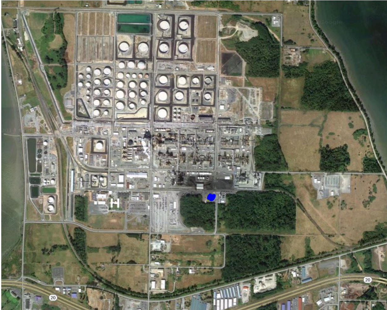
Figure 1-1 A view of the Matheson Tri-Gas facilities (position marked by blue dot), with the PSR refinery to the north (photo from google maps, accessed on 12/12/2014).
