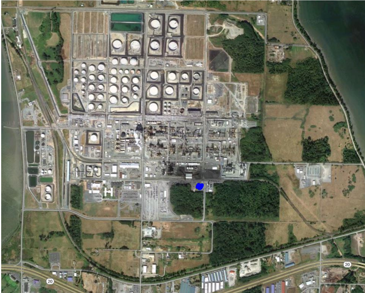
Figure 1-1 A view of the Matheson Tri-Gas facilities (position marked by blue dot), with the PSR refinery to the north (photo from google maps, accessed on 12/12/2014).
