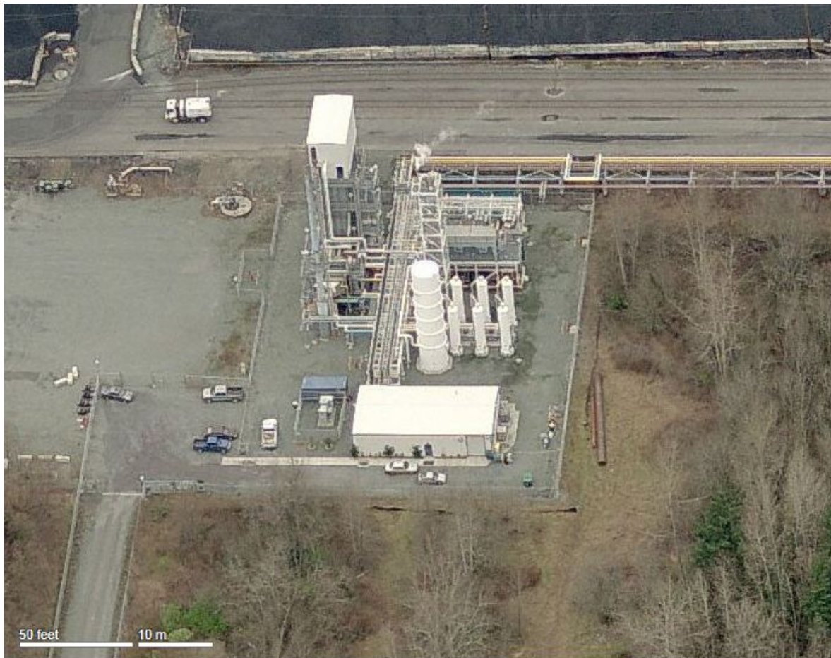
Figure 2-1 An aerial photograph showing the Air Liquide facilities at Anacortes, WA (photo from bing.com).
